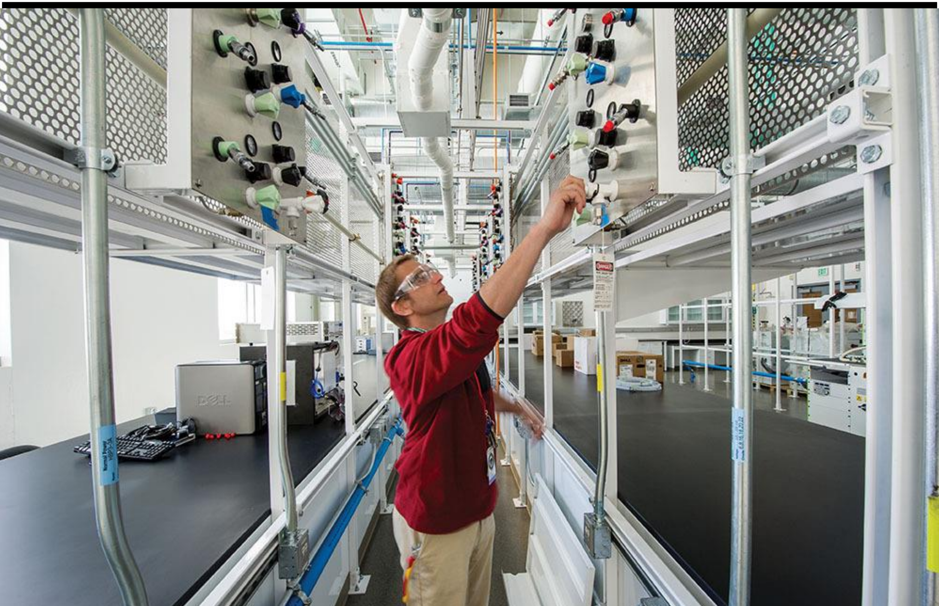
NREL researcher works in the gas manifold corridor for cell testing in the Fuel Cell Test and Development Laboratory
